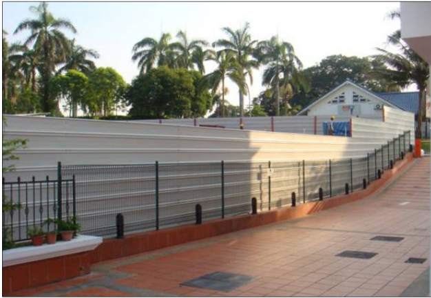
Photo 3.3.1c: Hoardings are maintained in good and clean condition through regular maintenance.
