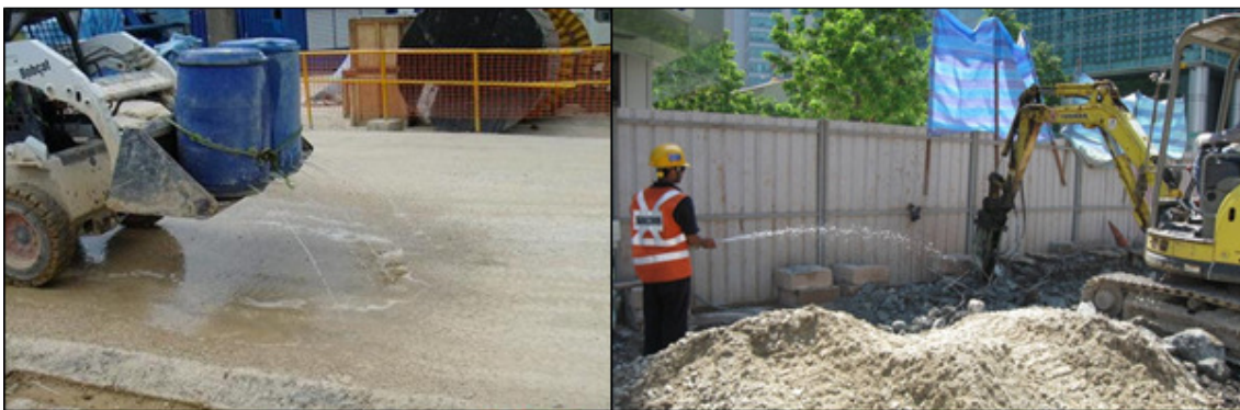
Photo 2.5.2b: Spraying water on site access roads and during hacking works will reduce dust generation. This is especially effective during dry days.
