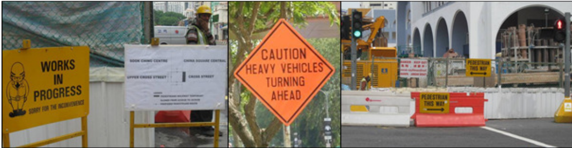
Photo 3.2.4a: Some examples of good signages around the construction site.
