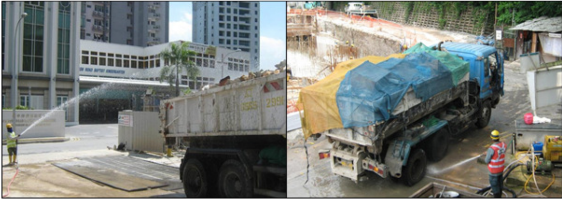
Photo 2.5.2c: Spray water to dampen dust generating materials and cover them properly during transportation.
