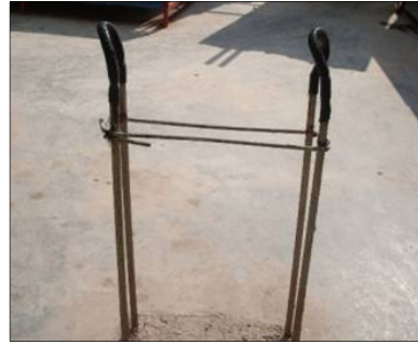
Photo 2.2.1e: Instead of throwing unwanted electrical wire hooks away, a builder can recycle them as rebar protectors on site.
