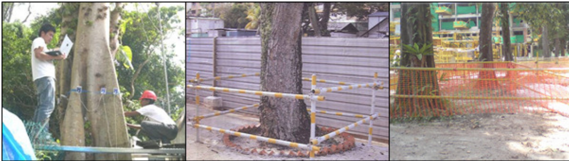
Photo 4.2.1b: The conservation of trees on site helps preserve the environment and provides shade and greenery for site staff. Specialists may need to be employed to monitor and recommend ways to preserve the health of the trees.
