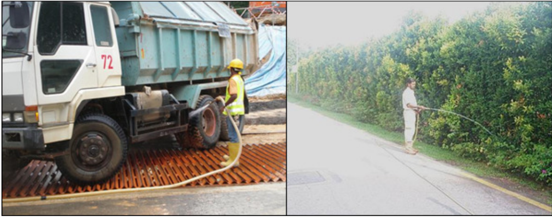
Photo 2.4.2c: Recycled water used for washing vehicles at washing bay and watering plants.
