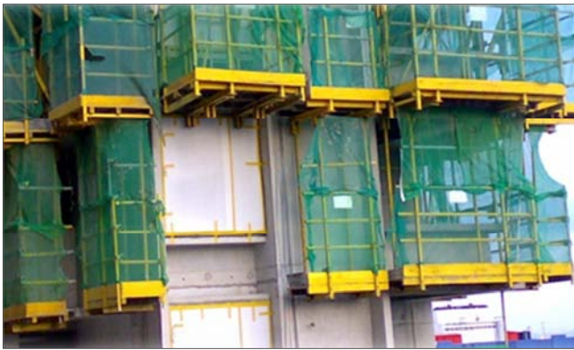
Photo 2.2.3d: The climbing cage system results in reduction of use of scaffolding.
