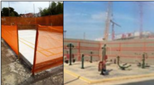
Photo 3.6.2c: Recreational facilities such as badminton courts and gym encourage leisure activities and cohesion among site personnel.
