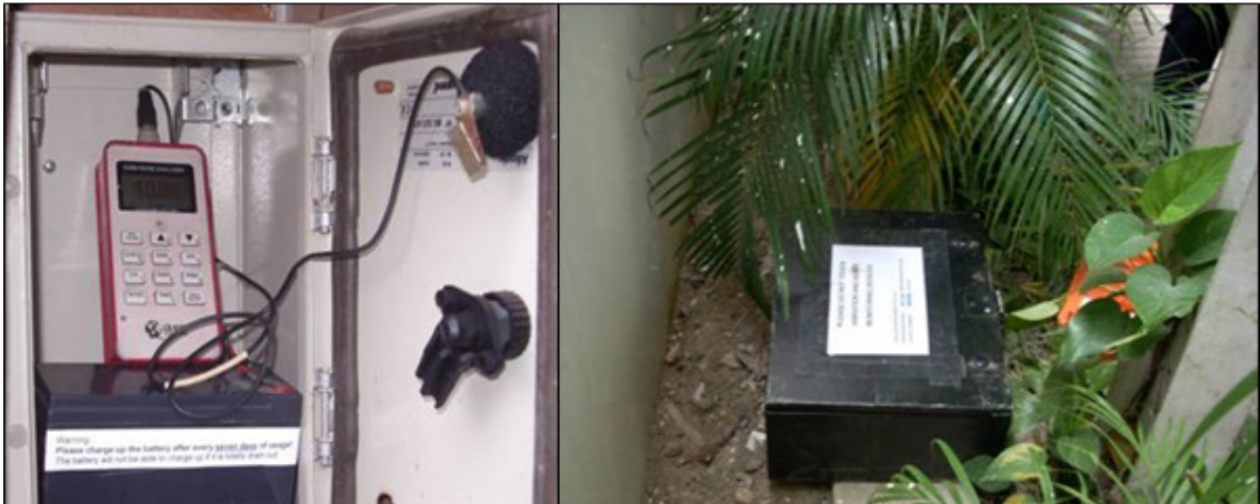
Photo 3.4.8a: Noise and vibration meters are installed for monitoring purpose.
