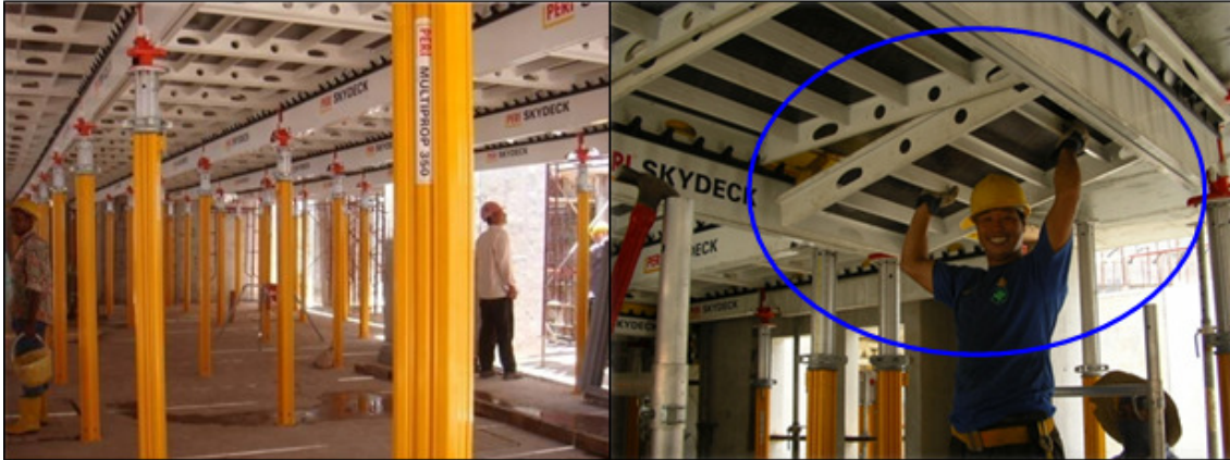
Photo 2.2.3a: The Integrated Modular Formwork is highly recyclable and requires less manpower to install and dismantle.
