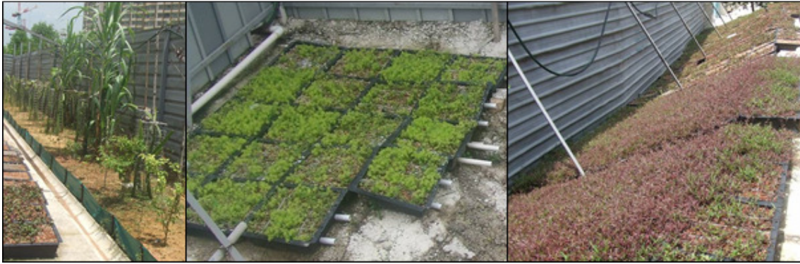
Photo 4.2.1c: Where space is available, plants and flowers can be planted extensively to beautify the site environment. These plants can also double up as erosion control measures to enhance the quality of water discharged out of the site.
