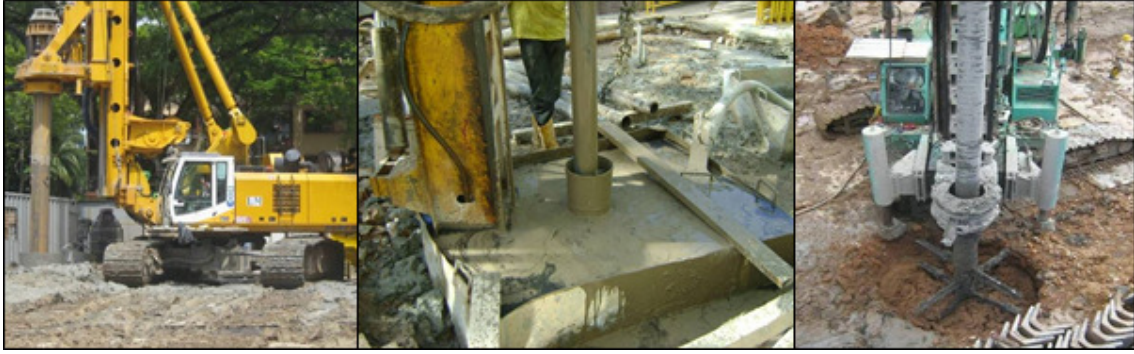
Photo 3.4.7c: Proper selection of piling system will mitigate noise and vibration felt by surrounding residents.
