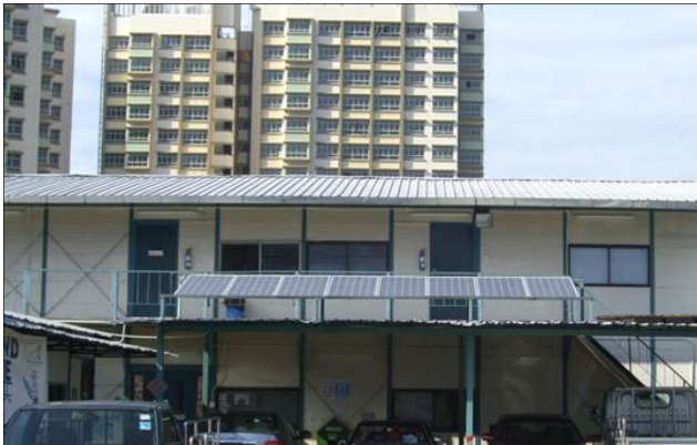
Photo 2.3.3a: Use of solar panels to help power the site office.
