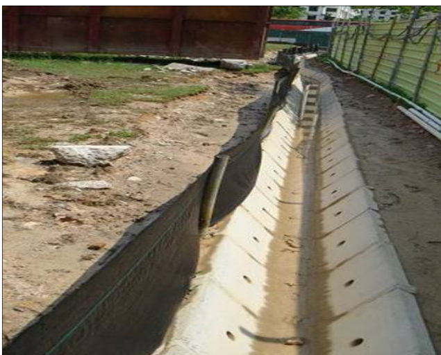
Photo 2.2.4a: Precast drains can use recycled aggregates and is popular among builders.
