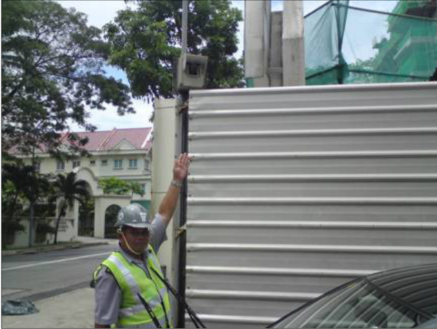
Photo 3.5.4a: CCTV can be used by the builder to enhance the security on site and minimize security concerns of neighbouring residents.
