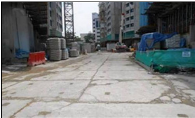
Photo 3.6.1b: A clean and conducive worksite can be created with the use of precast pavement.
