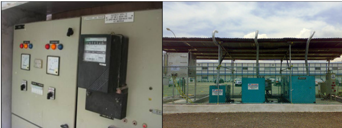
Photo 2.3.4a: Energy usage can be optimized through good management of alternating use of AC Grid power supply and diesel powered generators.
