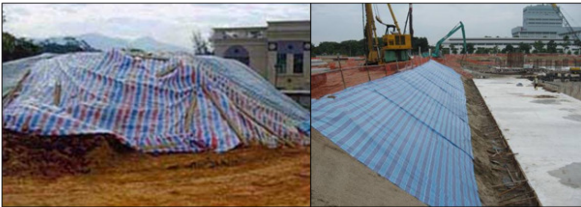
Photo 2.5.2a: Covering stock piles with sheets help to mitigate dust generation on site.
