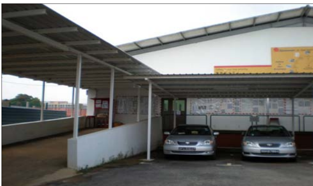
Photo 3.2.2c: A ramp has also been built near the site office.
