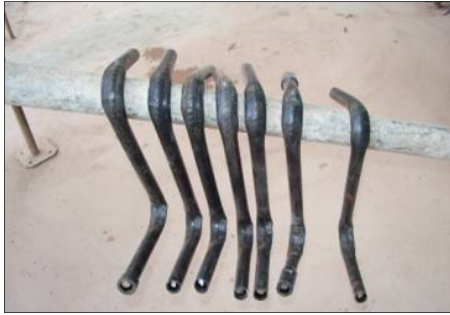
Photo 2.2.1e: Instead of throwing unwanted electrical wire hooks away, a builder can recycle them as rebar protectors on site.
