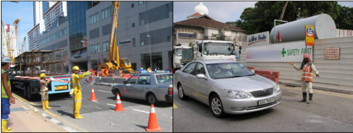
Photo 3.2.3a: The traffic controller guides traffic during concreting operations or materials delivery.
