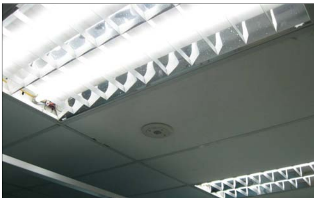
Photo 4.1.1f: Combining use of energy efficient T5 lightings and motion sensors can greatly reduce energy consumption in the site office.
