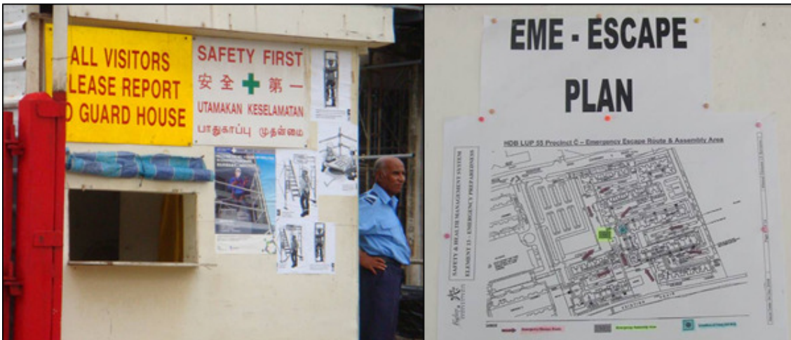
Photo 3.3.4a: Safety information and emergency evacuation routes are essential items to display to both staff and visitors on the site.
