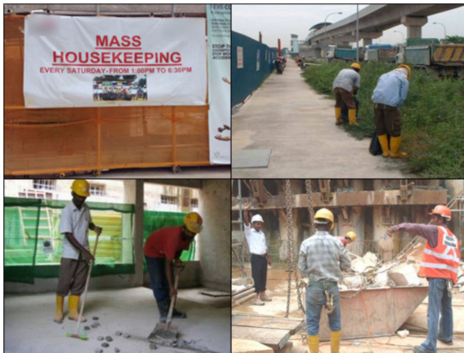
Photo 2.5.1a: A good housekeeping program will ensure all subcontractors adopt good housekeeping practices.
