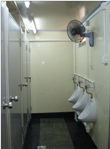
Photo 2.4.2b: Recycled water is commonly used for flushing toilets on site.
