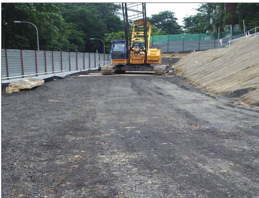
Photo 2.2.1d: Milled waste is recycled to cover access road on site. This practice greatly reduces environmental dust pollution generated on site.
