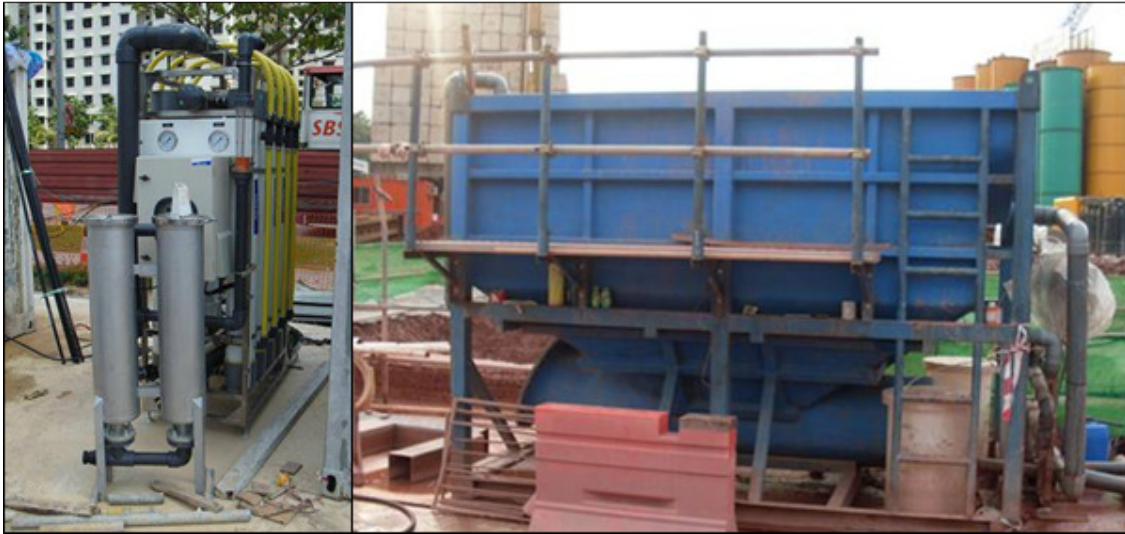
Photo 2.4.2a: Water treatment & recycling plant that utilize membrane (left) and chemical (right) technology.
