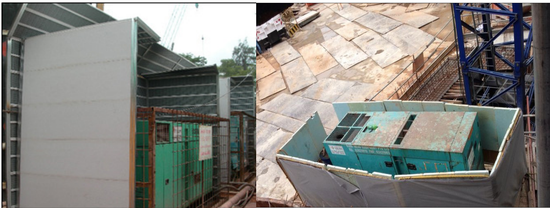
Photo 3.4.4b: Noise barrier panels around generators and machinery help to reduce the noise transmitted.
