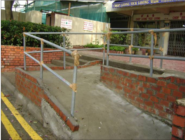
Photo 3.2.2a: A temporary ramp helps pedestrians at a walkway affected by construction works.
