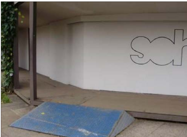
Photo 3.2.2b: A temporary ramp besides site hoardings is also useful to public users.
