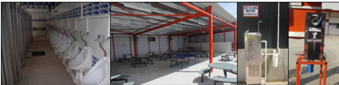
Photo 3.6.1c: Builder could show care for their site personnel's health by providing clean toilets, site canteen and hot and cold water points.
