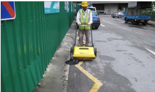
Photo 2.5.2d: Pavement sweeper is a useful equipment to clean up public roads or surrounding areas.
