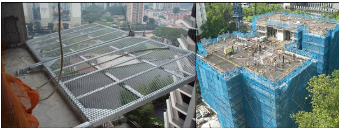
Photo 3.3.2a: The catch platform and safety netting work hand in hand to mitigate risk of falling debris.
