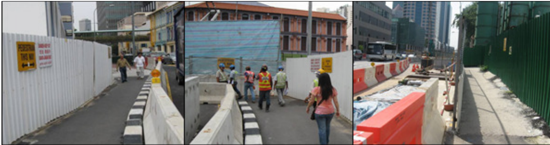
Photo 3.3.3a: Some examples of passageways provided around construction site.
