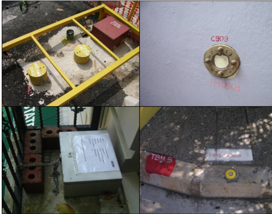
Photo 3.3.5a: Comprehensive monitoring of surrounding buildings can be done through the use of inclinometers, tilt meters, vibration meters and settlement markers.
