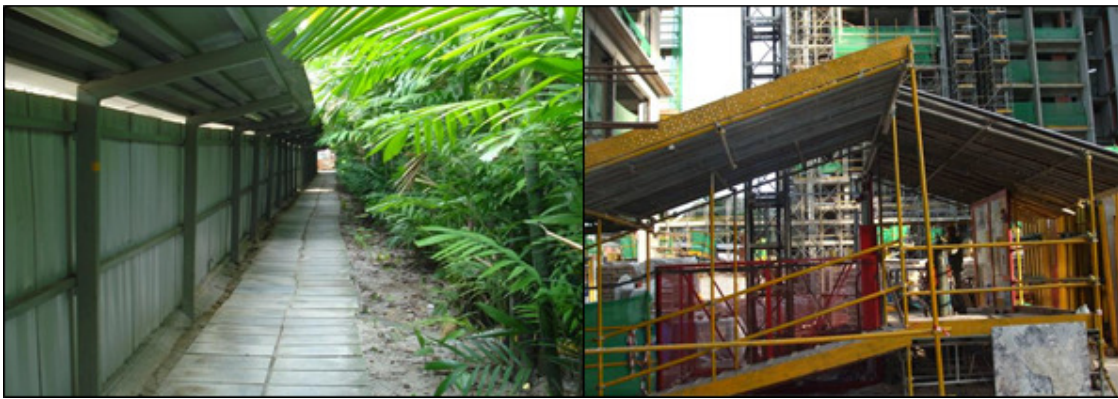
Photo 3.3.1a: Covered walkways around the perimeter as well as within the site provides protection and shelter.
