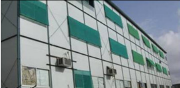
Photo 3.6.2a: Installation of nettings at on-site dormitory windows could aid in dust reduction and pest control of the rooms.
