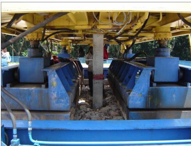
Photo 3.4.7b: Silent jack in piles greatly reduce noise and vibration produced.
