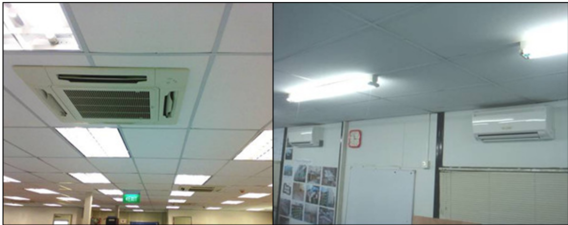
Photo 2.3.2b: Energy efficient air conditioning systems that comply with the Singapore's Energy Labeling Scheme helps to save energy in site office.
