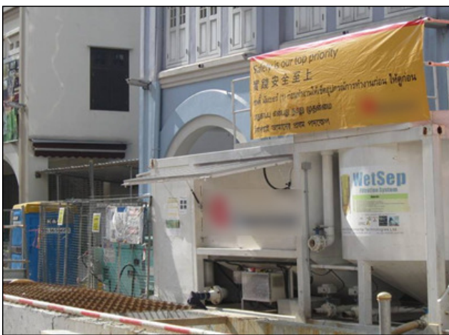
Photo 2.3.3c: Experimental use of solar cells to help power the water treatment plant.
