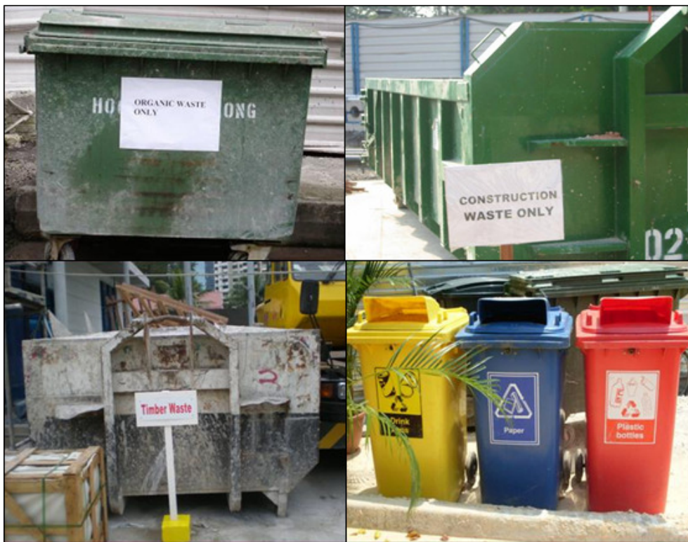
Photo 2.2.1a: The segregation of waste into construction, organic, or timber waste, metal cans, papers or plastic is the first step in Reduce/ Reuse/ Recycle.
