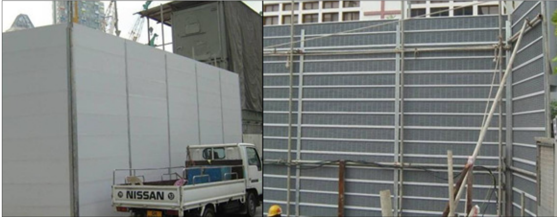
Photo 3.4.4d: High noise barriers can help reduce noise transmitted from the construction site.
