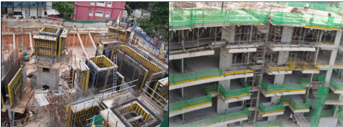
Photo 2.2.3b: The jump form and table form result in reduction of use of timber formwork.
