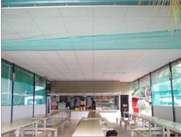
Photo 4.2.1f: Netting and false ceiling for canteen area ensure staff and workers can rest and eat in a cooler and dust free environment.
