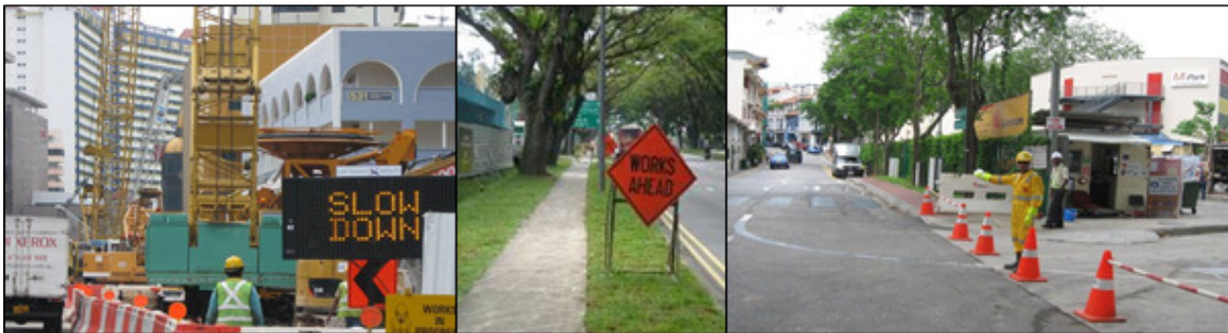
Photo 3.2.4b: Variable message sign (VMS) system complements role of traffic controller and usage of signages. This helps to minimize inconvenience to the public.
