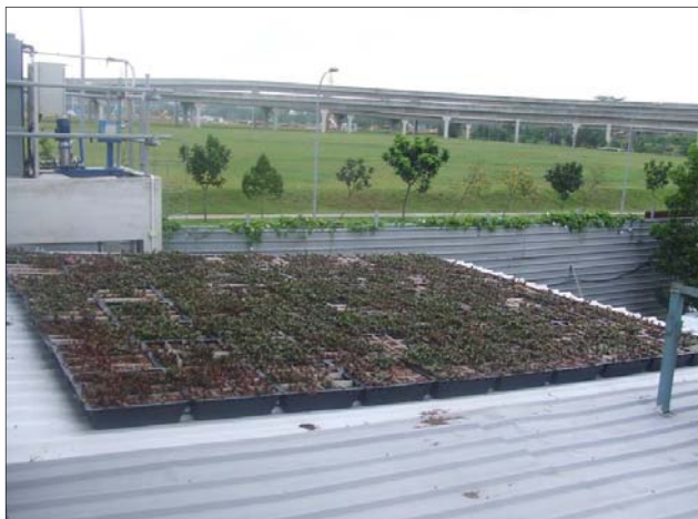
Photo 4.2.1d: A small roof garden above site office helps to cool the office.
