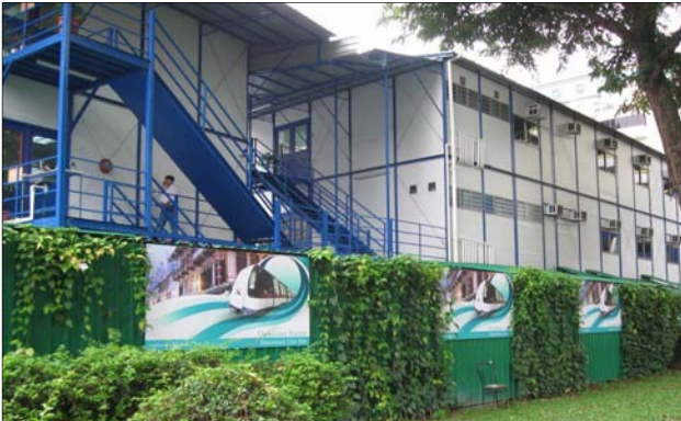
Photo 4.2.1a: The greening of hoardings not only builds a conducive working environment for staff and workers, it also portrays a positive image to the public.
