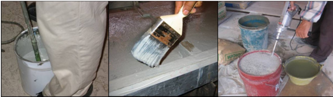
Photo 2.4.2d: Recycled water used for grouting, waterproofing and tiling works.
