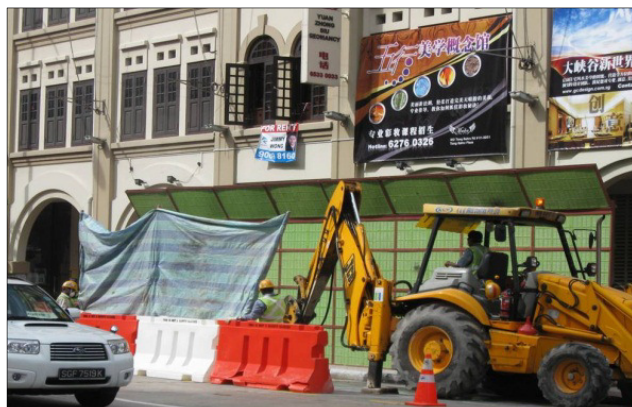
Photo 3.4.4c: Use of movable noise barriers can also reduce the noise transmitted from machinery.
