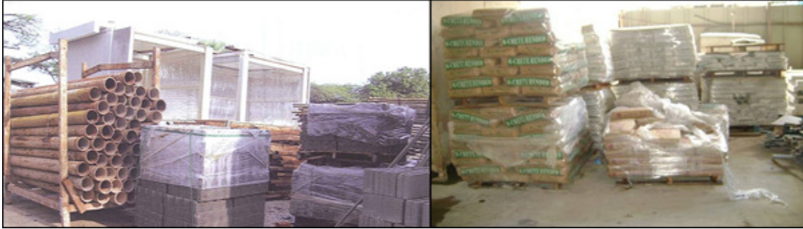
Photo 2.5.1b: Designated storage spaces allow materials to be properly stored on site.
