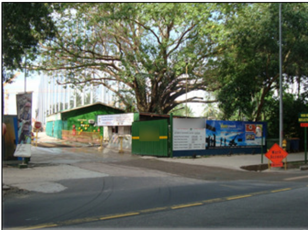
Photo 3.2.1a: A clean and unobstructed site entrance portrays a positive image of the builder to the public.
