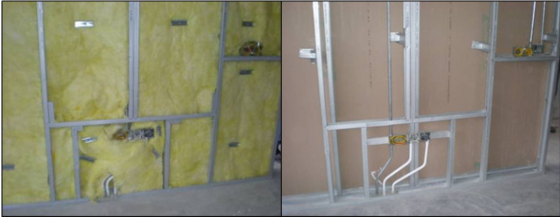
Photo 2.2.3c: Usage of drywalls will reduce masonry works on site.
