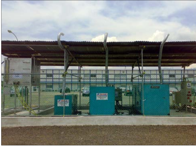
Photo 4.1.1d: The bigger capacity generators can be used in the day when the energy consumption is higher while the smaller capacity generator can be used at night when energy consumption is lower. This will optimize the usage of diesel and results in cost savings.
