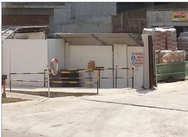
Photo 3.2.3b: A traffic mirror can be used to show blind spot.
